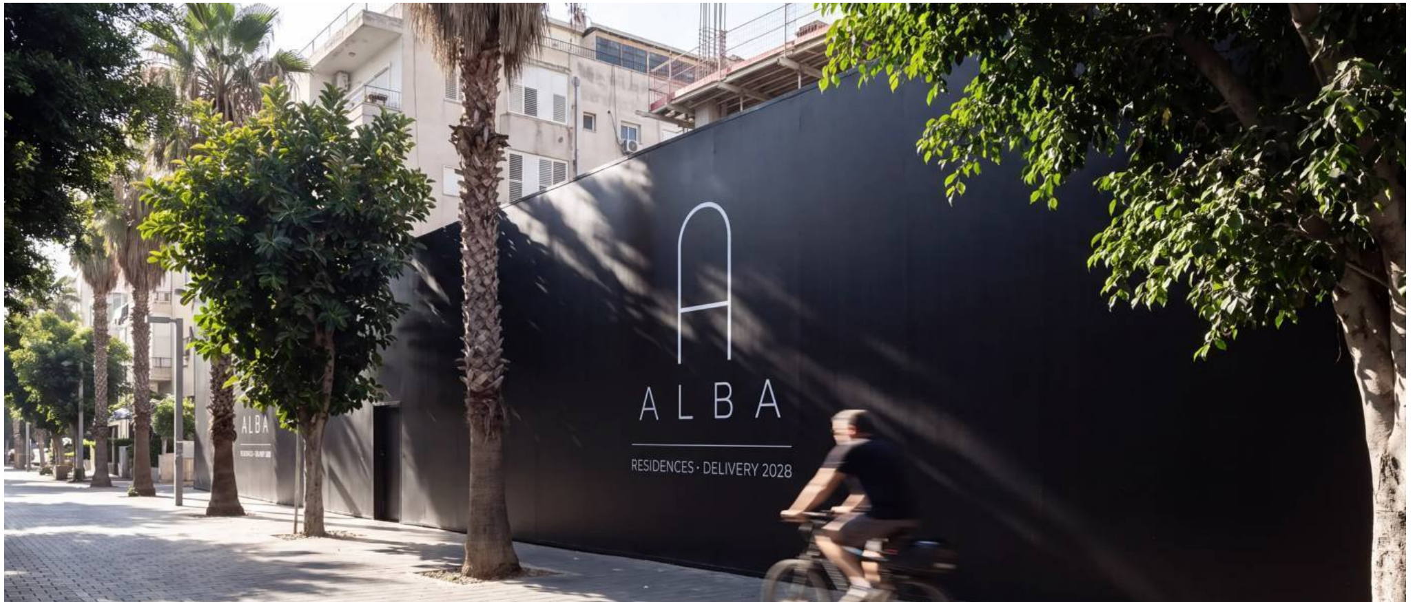
SITE HOARDING, ROTHSCHILD BOULEVARD
